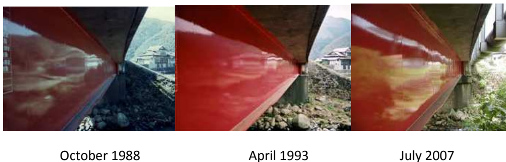
Figure 6: Photos of the Tokiwa Bridge Over 21 Years
